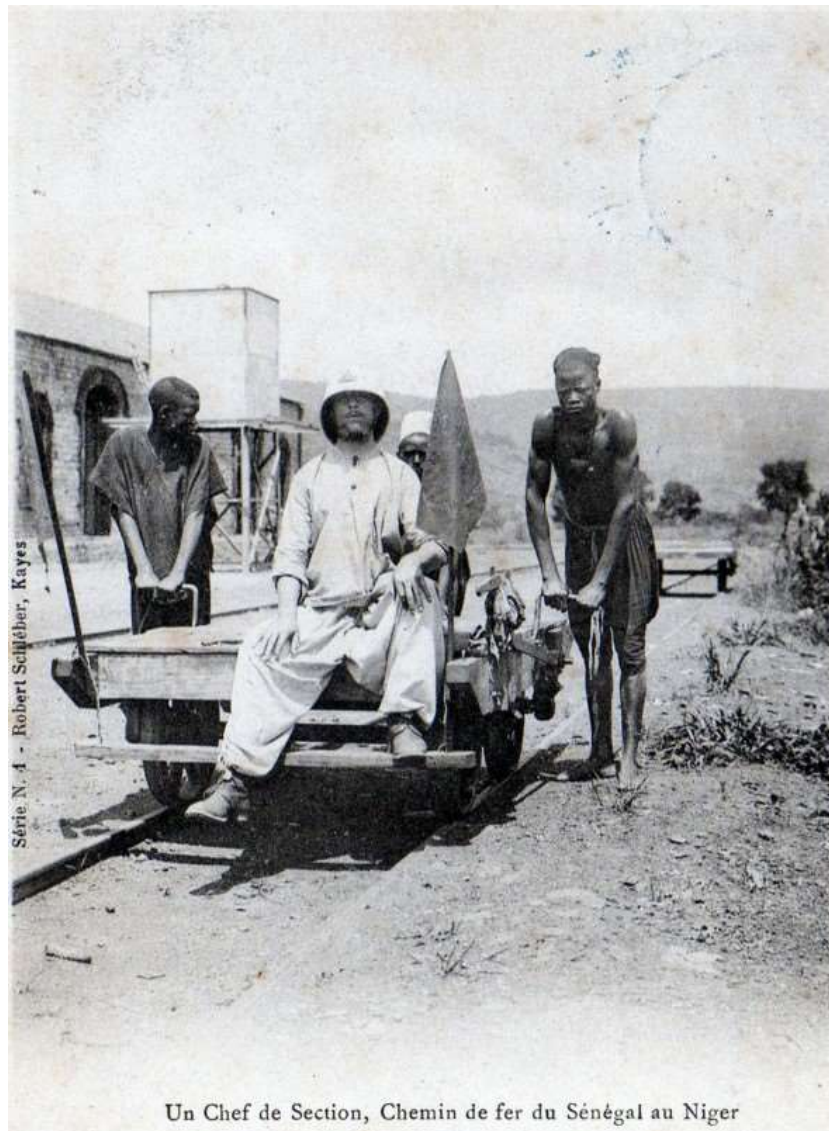
Un Chef de Section, Chemin de fer du Sénégal au Niger Série N. 4 - Robert Schléber, Kayes A Section Chief in the building of the Dakar–Niger Railway, pushed by African workers, Kayes, Mali, 1904 - Robert Schléber, Kayes - Collection Jean-Pierre Vergez-Larrouy (1903).
